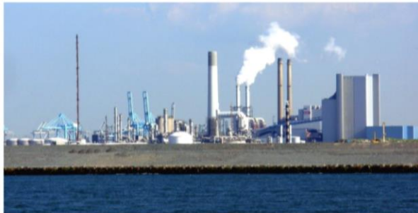
The Uniper plant in Rotterdam (Credit: Wikimedia Commons)
