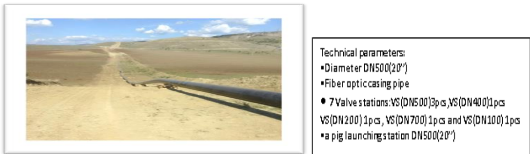
Picture 4. Construction of Lot1'
