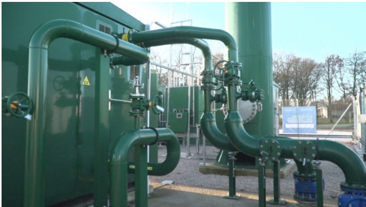
Figure 37 Gas grid injection of hydrogen as part of the HyDeploy project
