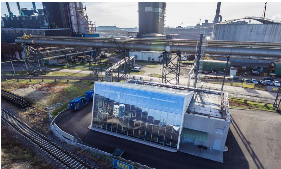
Figure 36 The Voestalpine steel production plant in Linz, Austria
