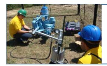
The main task is to search for and measure natural gas leaks from GTS equipment, as well as to eliminate leaks by filling the problematic fittings with gas-sealing mastics.
