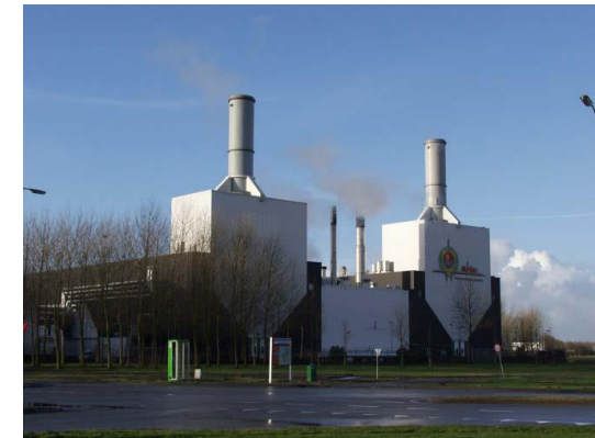
Combined Heat and Power Plant
