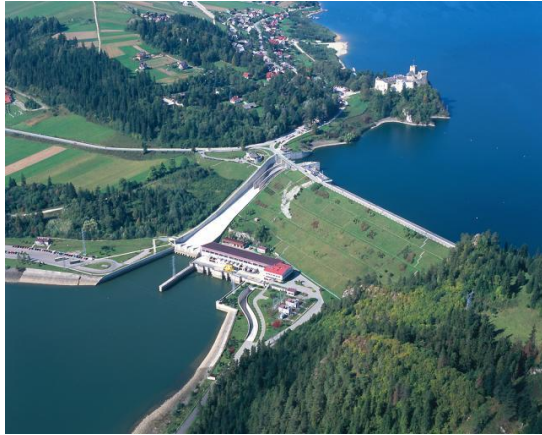
Hydro Power Plant
