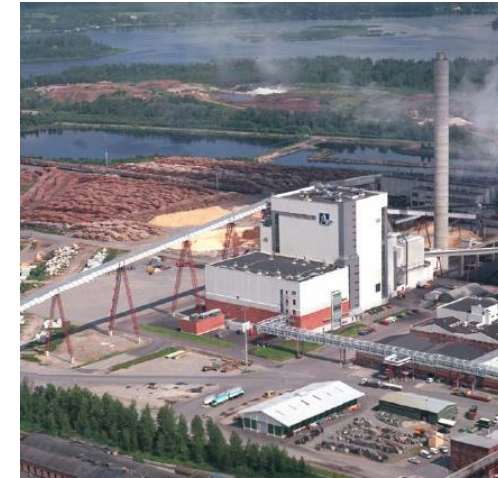
Biomass Power Plant
