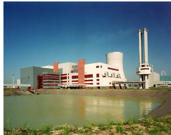
Waste to Energy Plant
