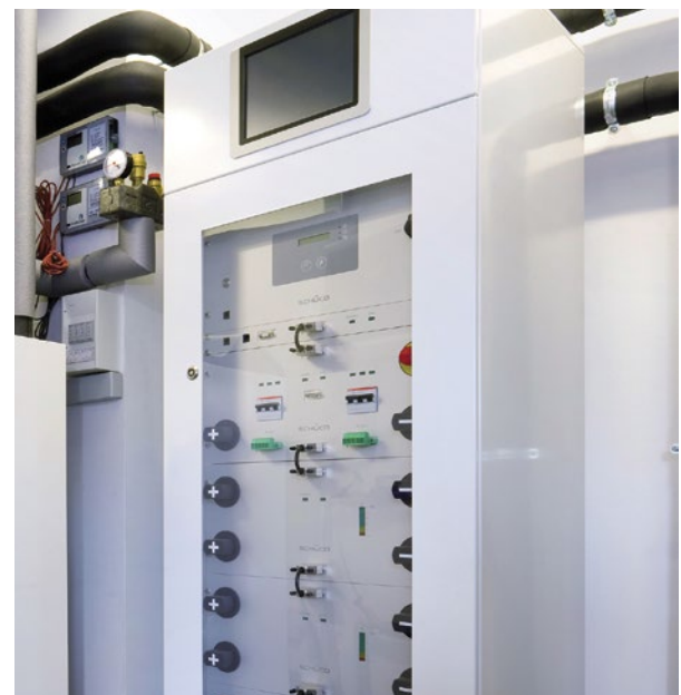
Battery storage, 13.2 kilowatt hours
