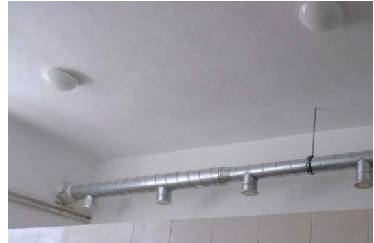
Figure 6: New surface mounted luminaries in toilets
