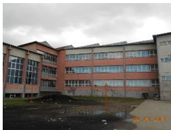
Figure 14: Rear & Side Facade
