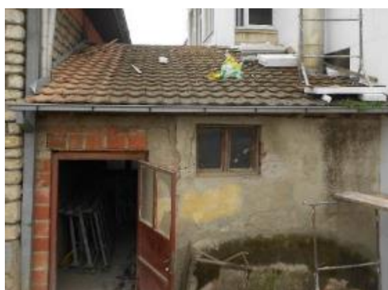
Figure 3: Existing boiler room
