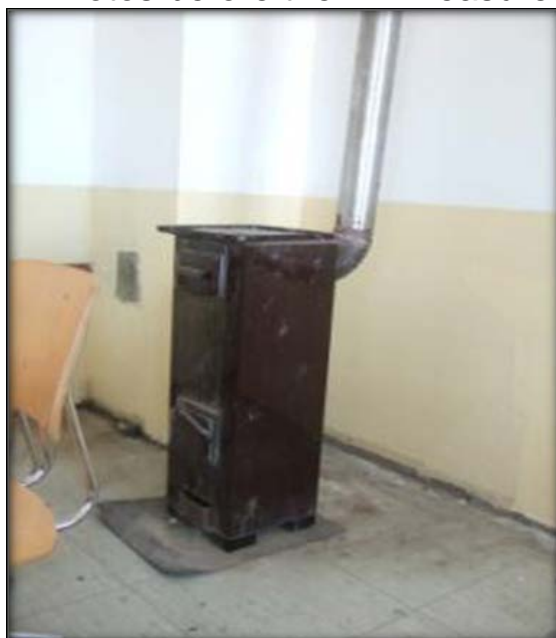
Photos before the EE measures- Heating System with old system stove
