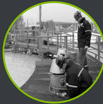
Storage Tank, LNG Emission Management
