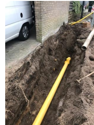
Pipelines (typ. 100mbar) + Service lines
