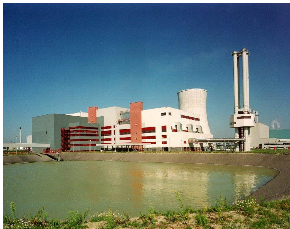
Waste to Energy Plant
