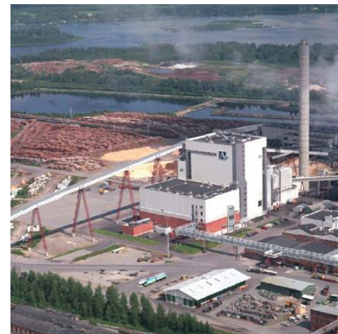
Biomass Power Plant
