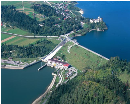
Hydro Power Plant
