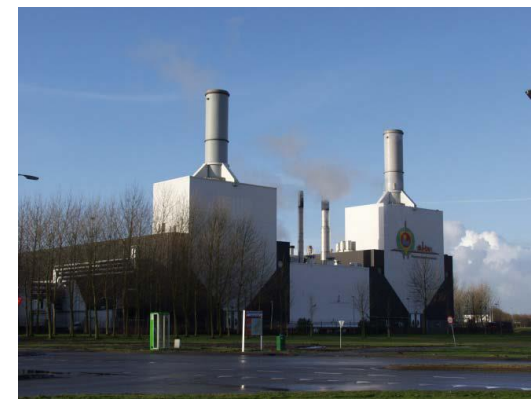
Combined Heat and Power Plant
