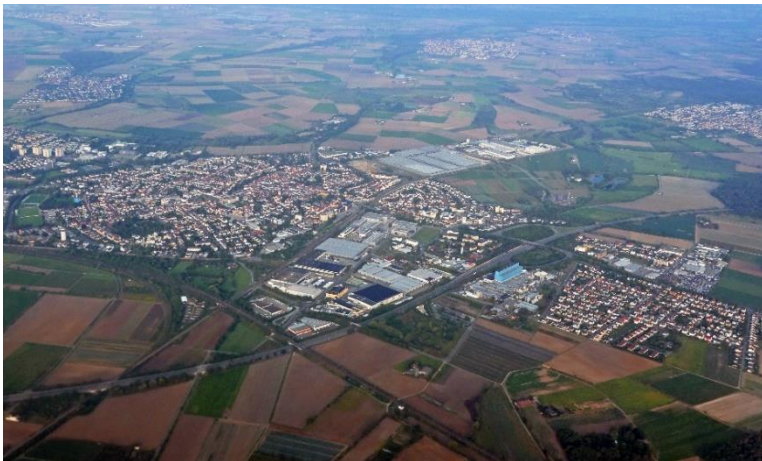
Geothermal project in Groß-Gerau (Germany)
