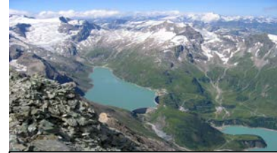
Optimisation, Water Value
