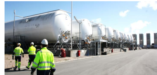
LNG reloading and bunkering station under construction in Klaipeda
