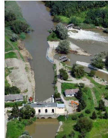
Hydro power plant
